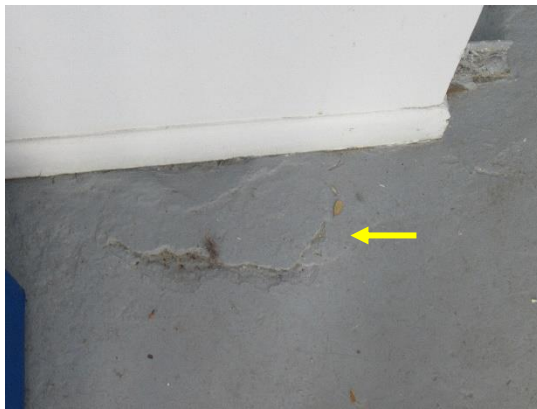
View of delaminated concrete in the laundry room.
