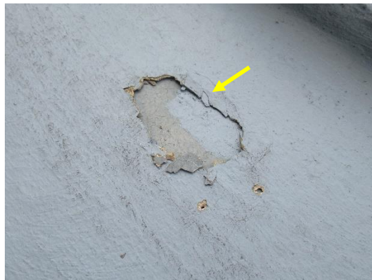
View of deteriorated coating on the breezeways.
