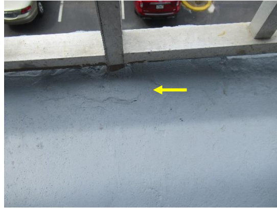
View of delaminated concrete on breezeway.
