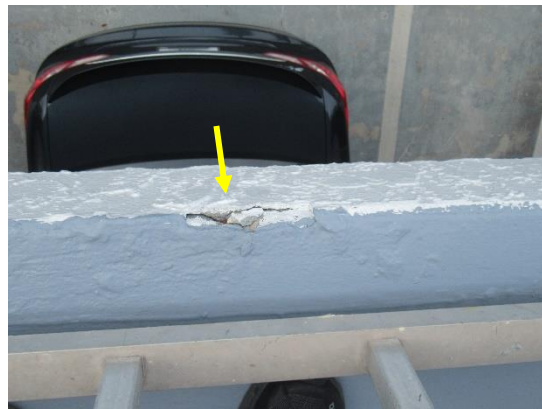
View of delaminated stucco on the breezeway edge.
