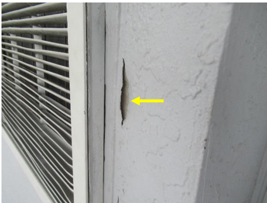
View of typical delaminated paint.
