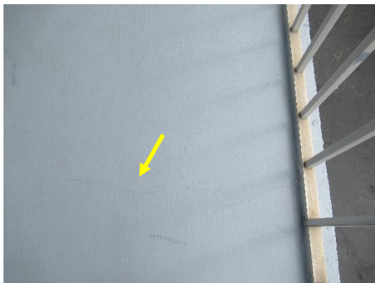
View of typical breezeway crack.
